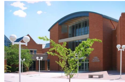
The Scott Center for the Fine and Performing Arts, the Hikel Business Training Center, and the Life Fitness Building opened in 2002.
